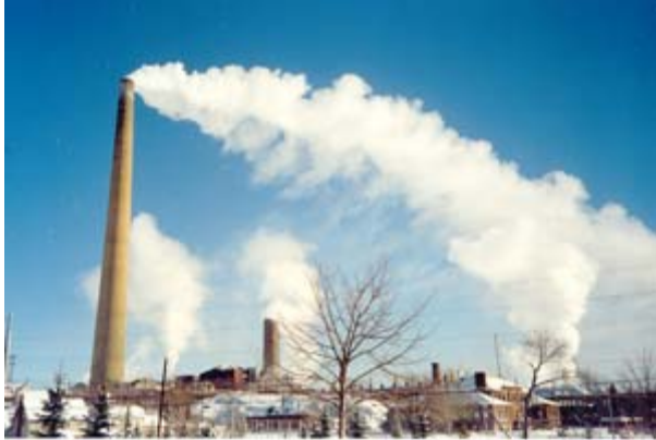
The VALE INCO "Superstack", located at Sudbury, Ontario
