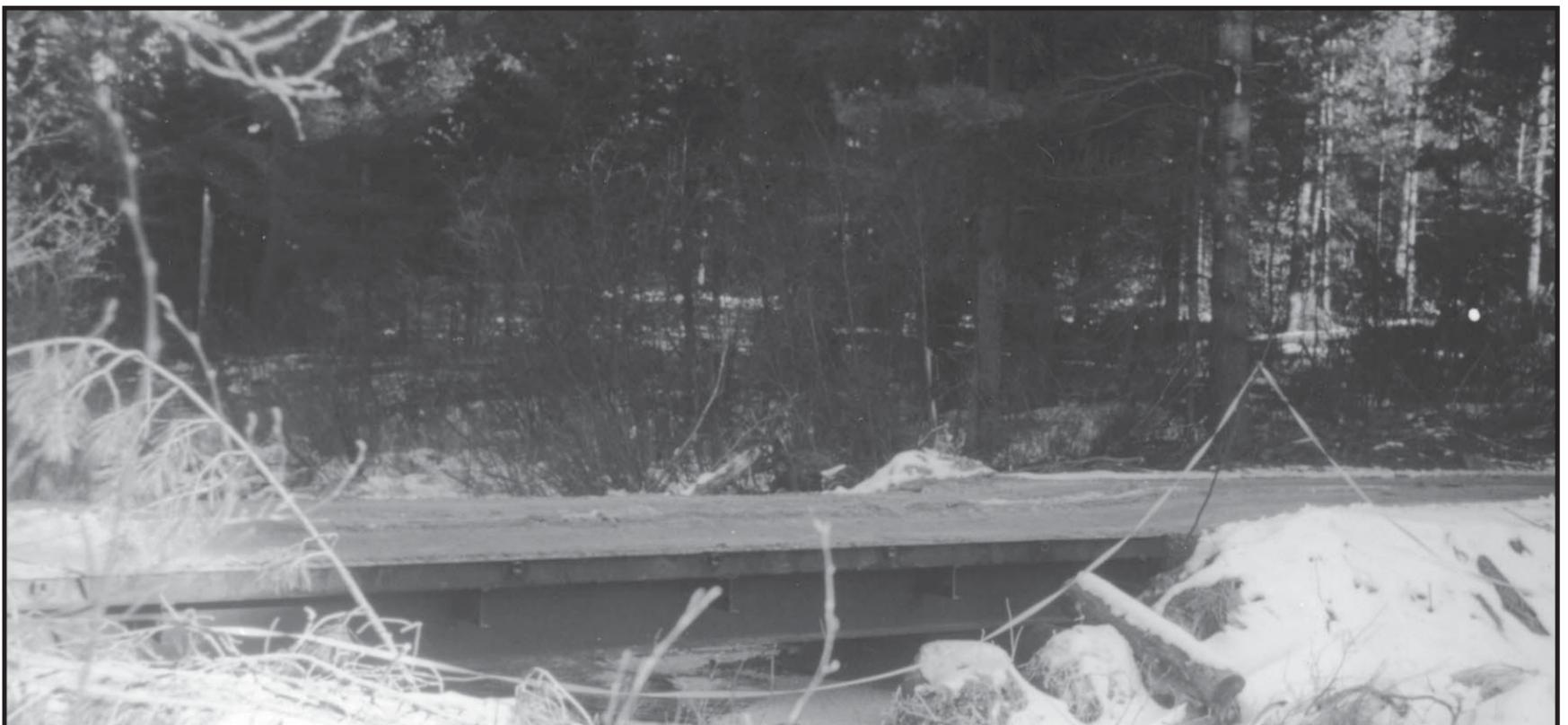
*This portable metal bridge, spanning a brook trout nursery creek, was fabricated for the Algonquin Forestry Authority, and can be removed for use elsewhere, with no resulting damage to the creek bed.*
